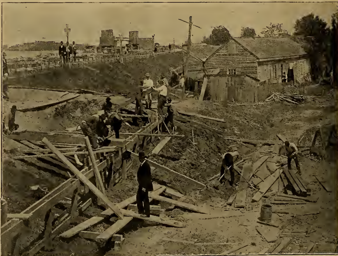
BRACING A WEAK LEVEE.
